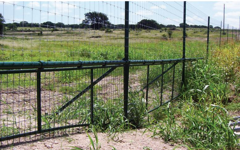
Fencing with water gaps Any of these materials make excellent water gap supports. Specifically, we recommend galvanized pipe or wood treated for use in high water situations. Remember to drive support posts into a sturdy place on the bank.
