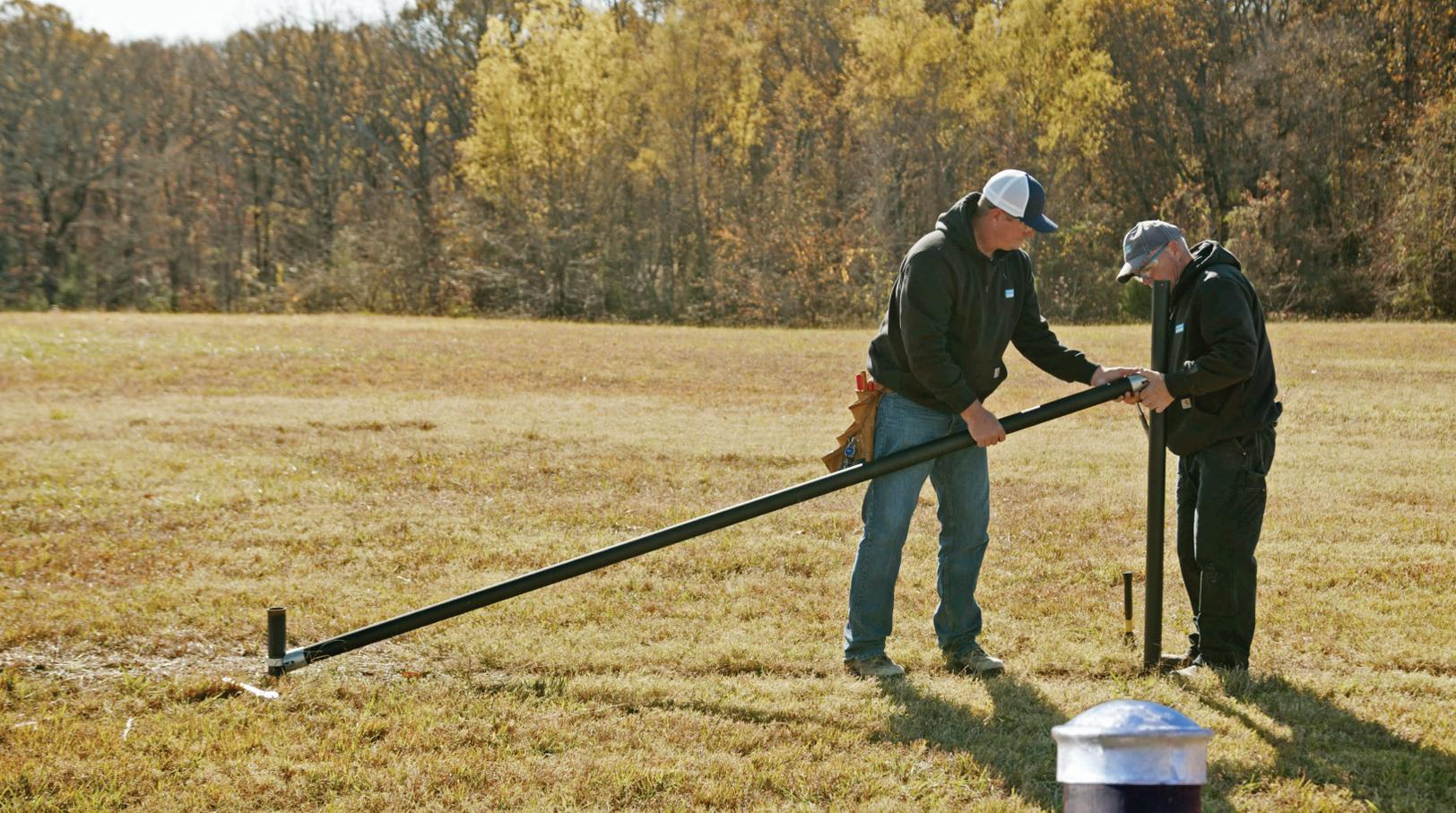
With uprights in and pipes cut, it can take as little as five minutes to connect an H style or N style brace or just 10 minutes for an HN style brace.
