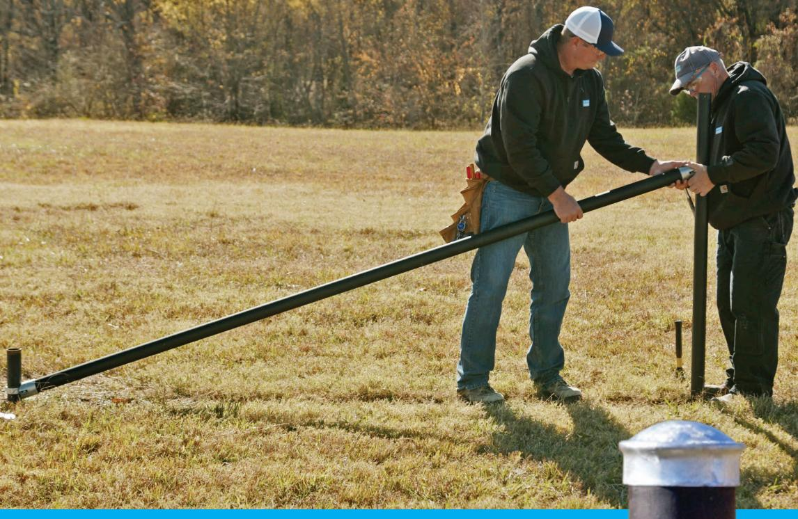
With uprights in and pipes cut, it can take as little as five minutes to connect an H style or N style brace or just 10 minutes for an HN style brace.
